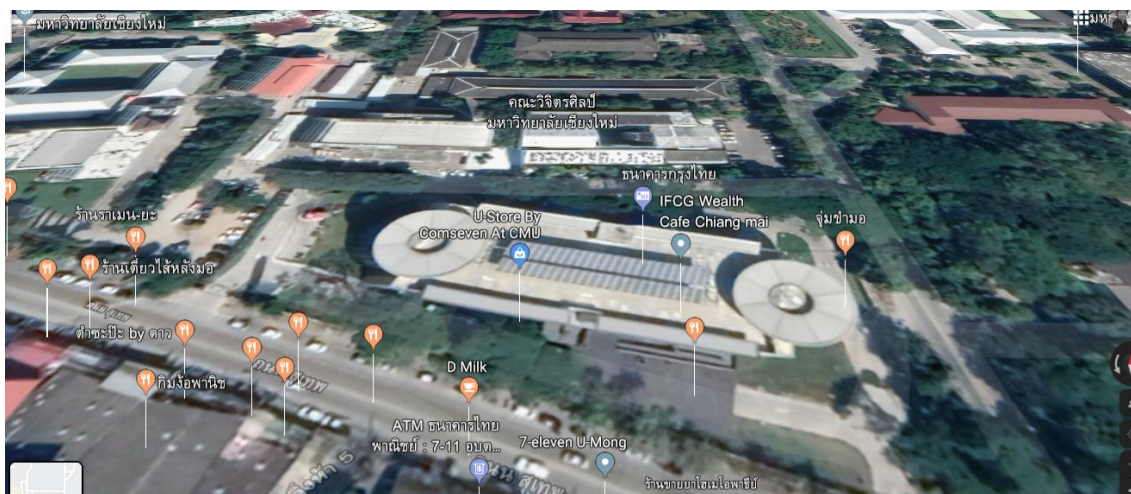
รูปที่ 2. 29 Solar rooftop in S1 building, CMU (Source: Google earth shot on 10 June 2018)
