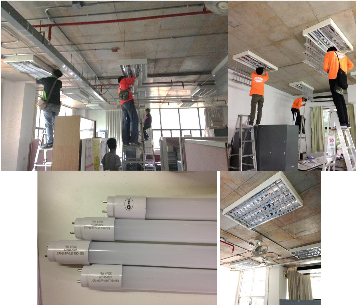
รูปที่ 2. 12 LED lighting fixtures are replacing conventional appliances (individual adjustment in all fixture)
