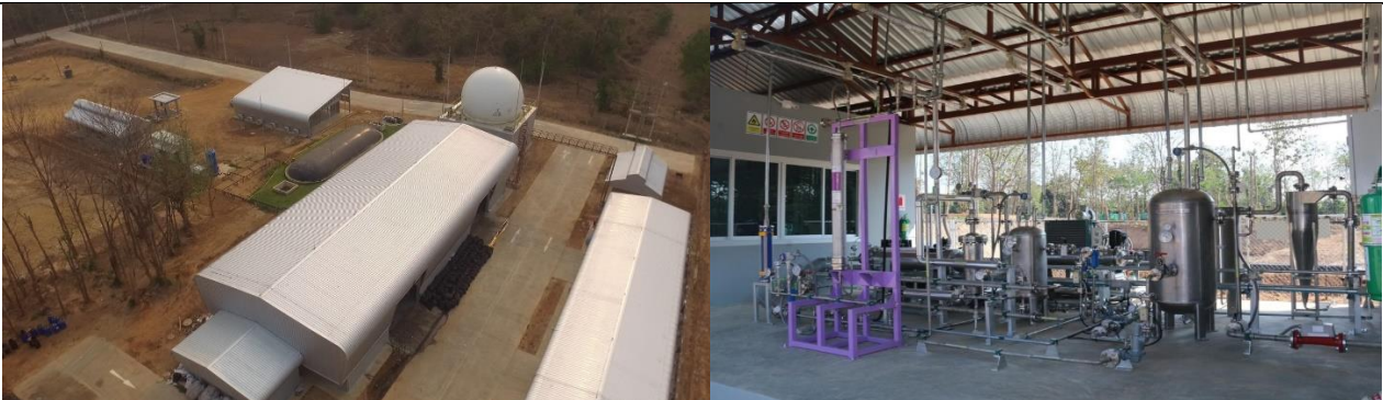
Integrated solid waste management plant (taken on 20 June 2018)
