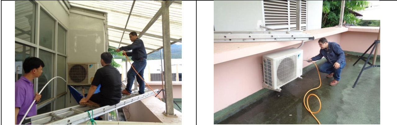
A/C cleaning in FACMU building (Source: shot on 7 Aug 2019)
