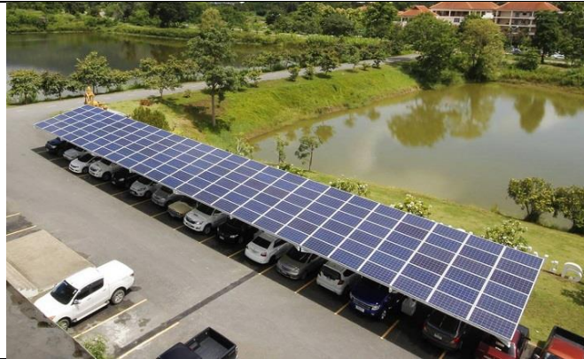
Example of Solar Roof (Energy Research and Development Institute – Nakornping)
