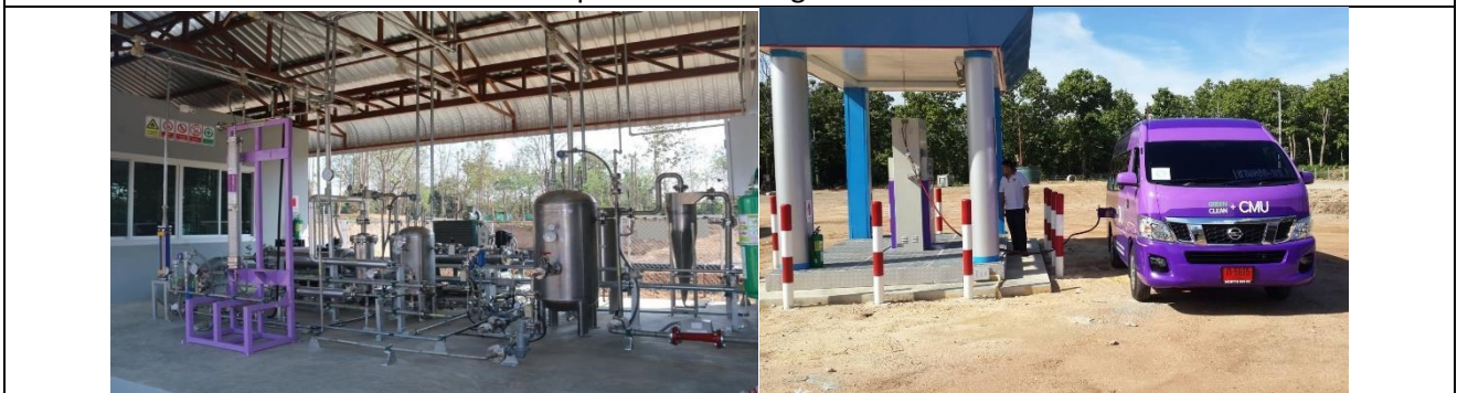
Garbage sorting machines (upper) Bio-gas testing instrument and CBG station (lower)
