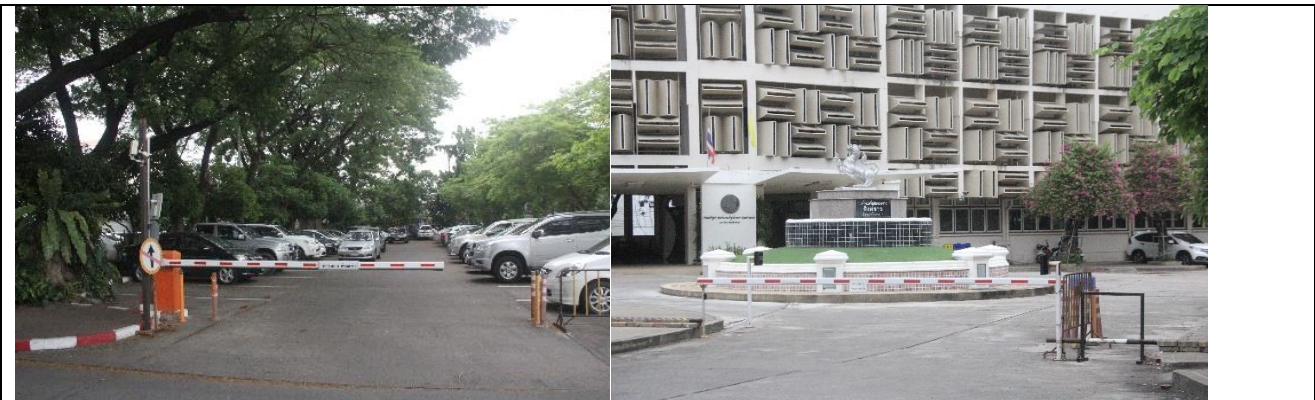
Examples of the use of automatic RFID enclosure systems at the Faculty of Medicine (left) and the Faculty of Political Sciences and Public Administration (right) (1)
