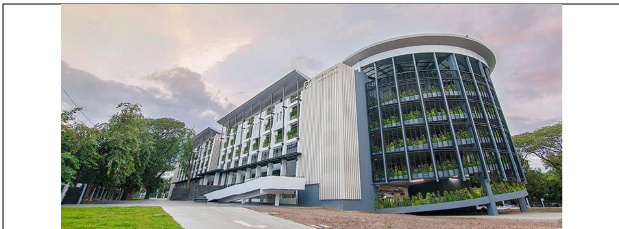
The S1 Building reuses the treated wastewater for vertical garden watering. (WT)
