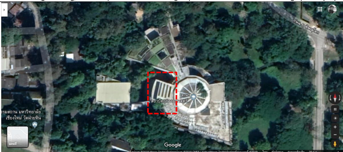
Solar rooftop on FACMU building [E1,E2]
