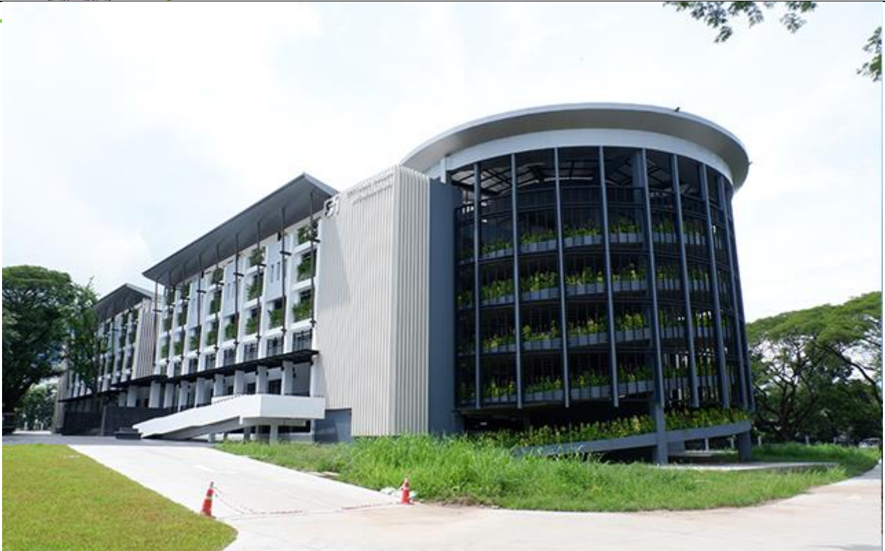
S1 Parking Building, an example of Smart Building implementation on Smart Parking system [B2]
