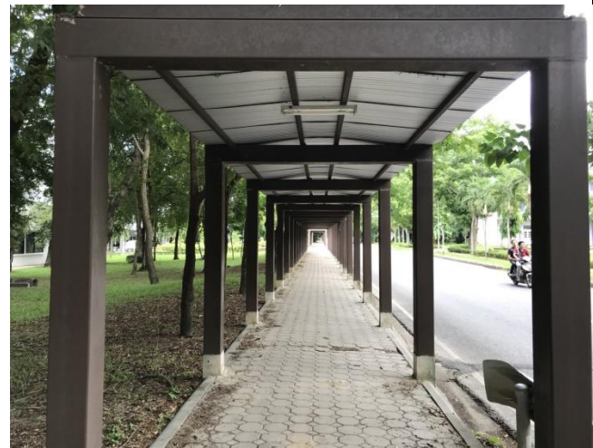
4) Covered walkways with lighting at night
