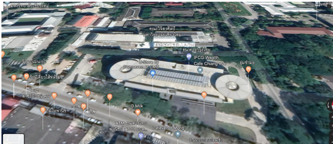
A solar rooftop system of S1 building, CMU (Source: Google earth, accessed on 10 June 2018)
