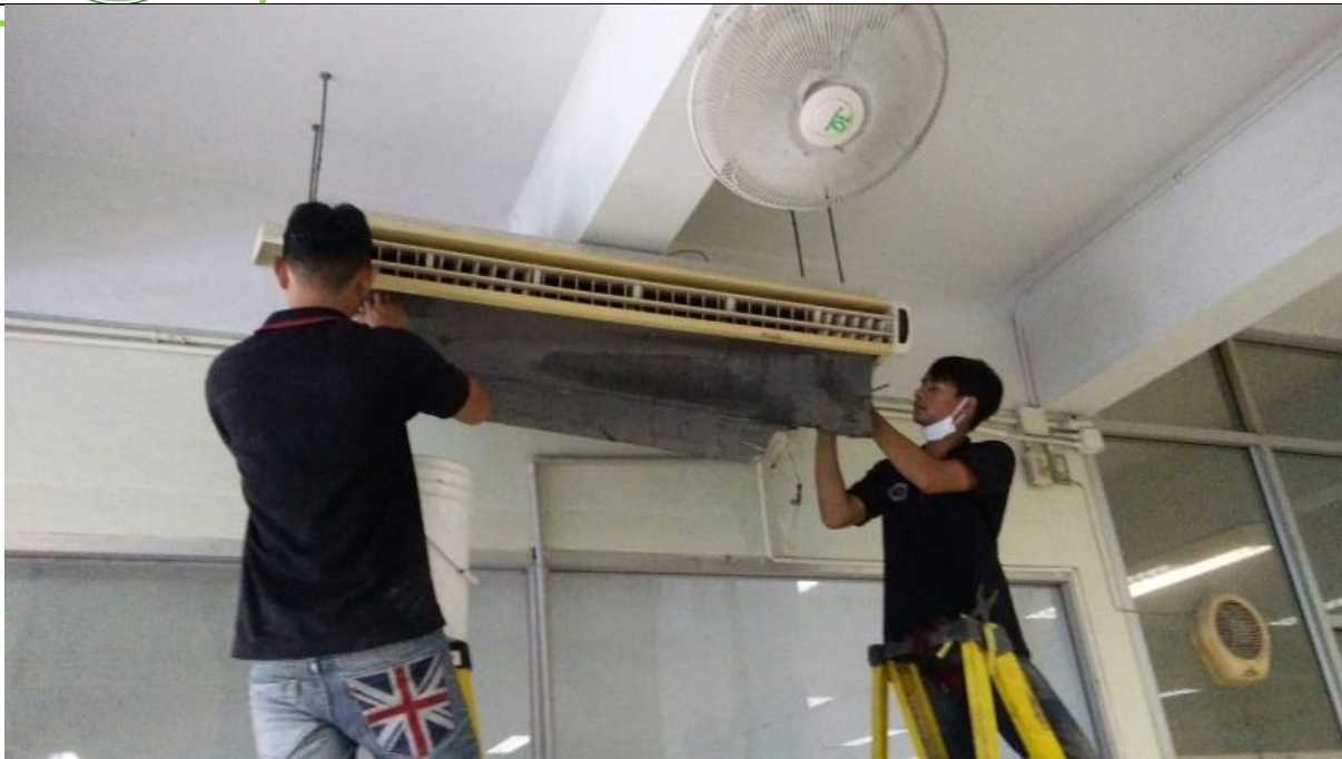
A/C cleaning in Faculty of Architecture Building. (Source: shot on 15 Feb 2018)
