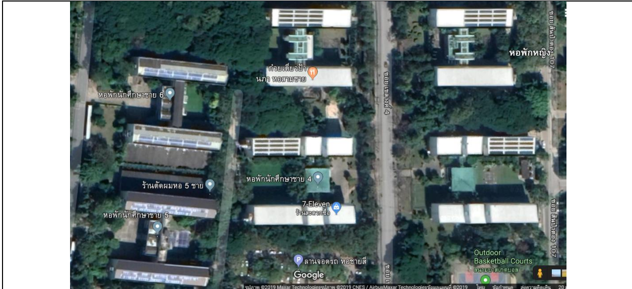
Solar rooftops on Domitory Buildings, CMU (Source: Google earth, accessed on 10 June 2018)
